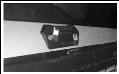
INSTALLED UPPER ANCHOR
